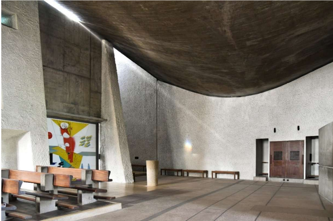
24. Le Corbusier, Notre-Dame du Haut , Ronchamp, South Chapel Entry with Hovering Ceiling
