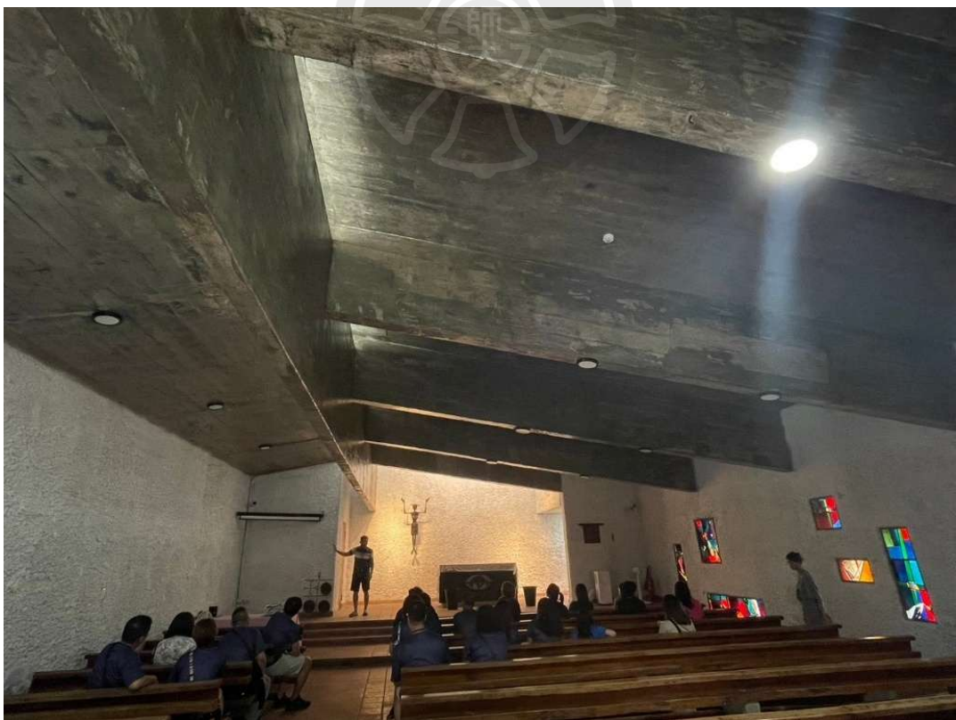
21. Justus Dahinden, Saint Joseph's Chapel of Kung-Tung , Western Portion of the Ceiling Supported by Four Transversal Concrete Fasciae
