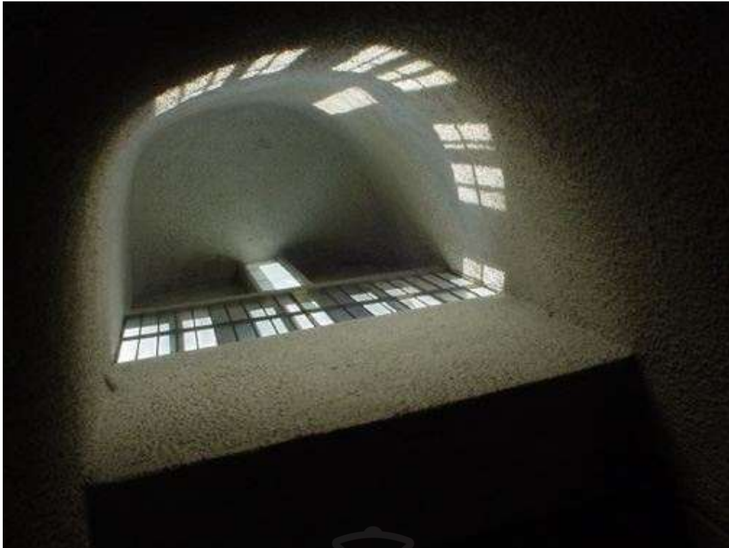
30. Le Corbusier, Notre-Dame du Haut , Ronchamp, Gunnite on the Walls with Sculptural Mass of the Vault
