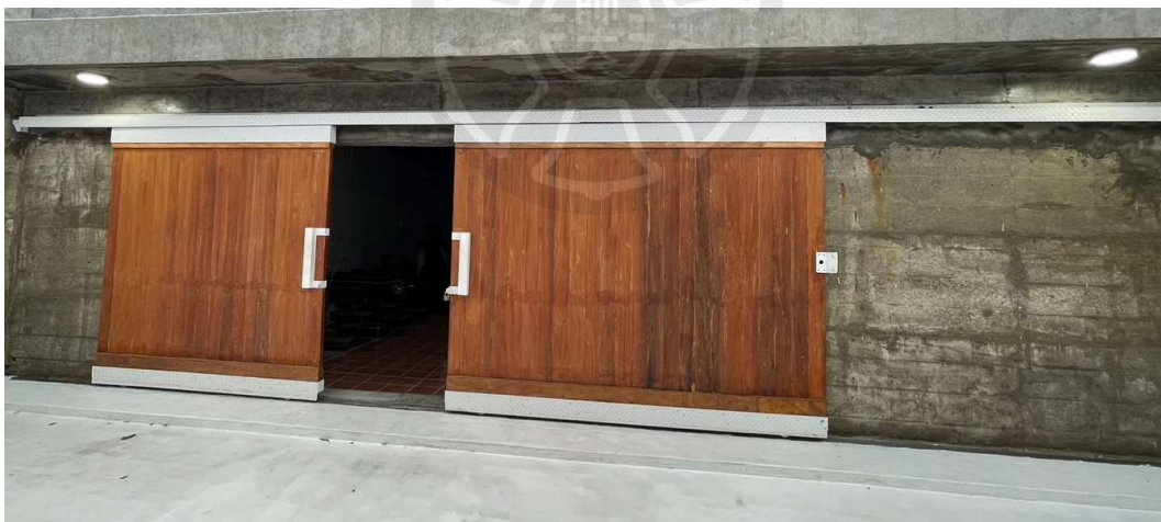
38. Justus Dahinden, Saint Joseph's Chapel , Taitung, Two Recessed Spotlights Above the Exterior Sliding Doors
