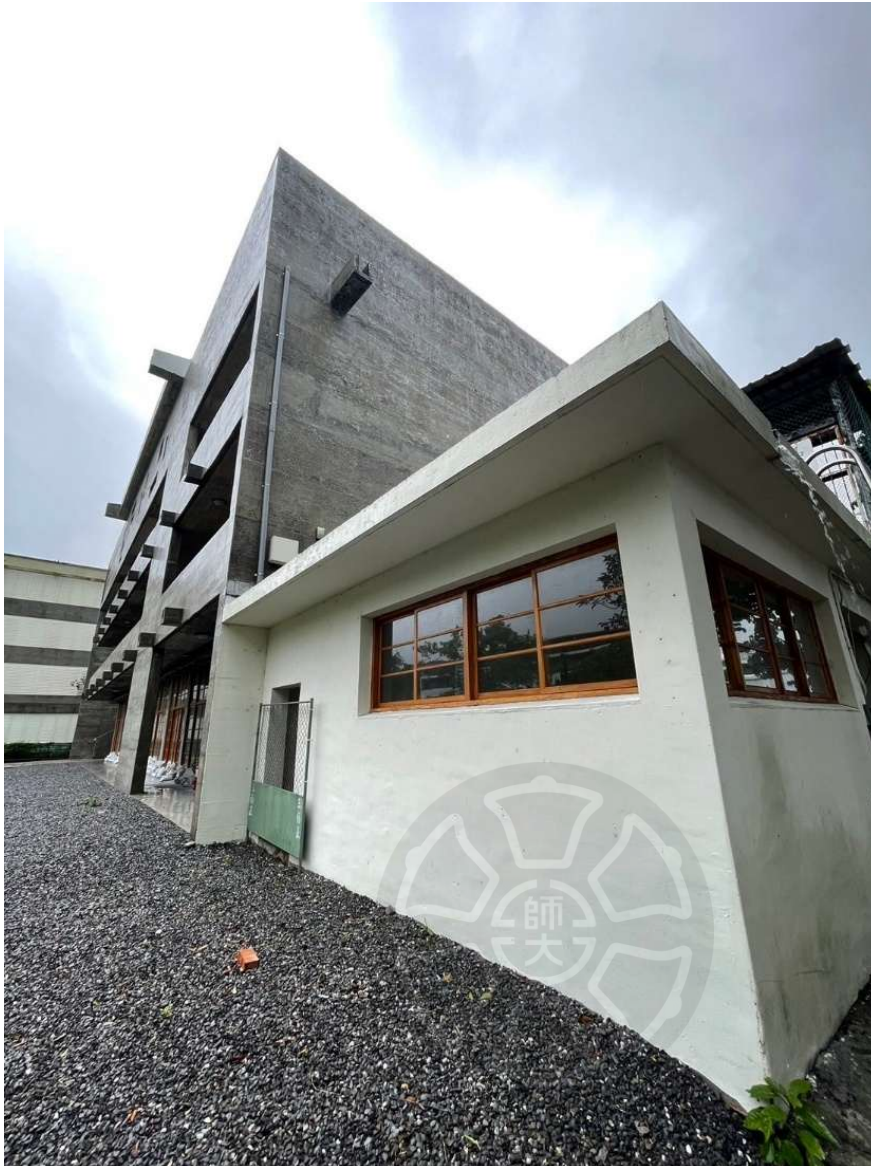
12. Justus Dahinden, Saint Joseph's Chapel of Kung-Tung , Side Room at the Southwest Corner
