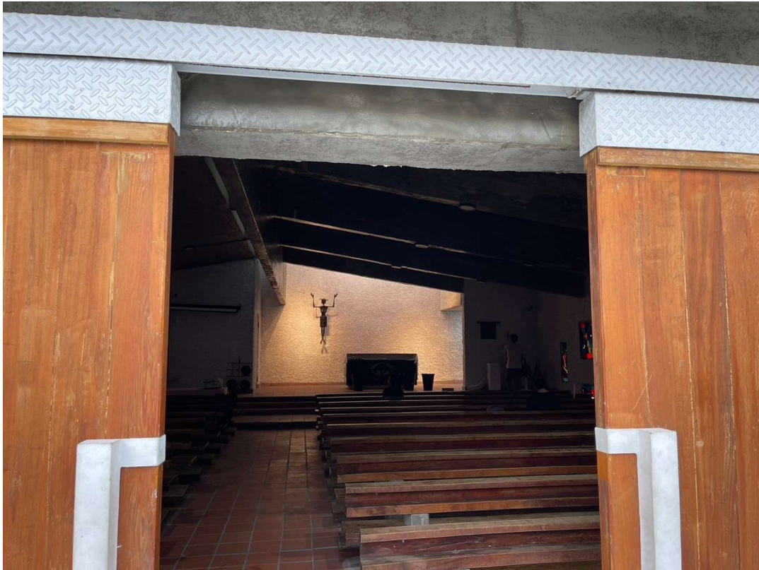
35. Justus Dahinden, Saint Joseph's Chapel of Kung-Tung , Chapel Entrance with Wooden Sliding Shutters on Metal Guides
